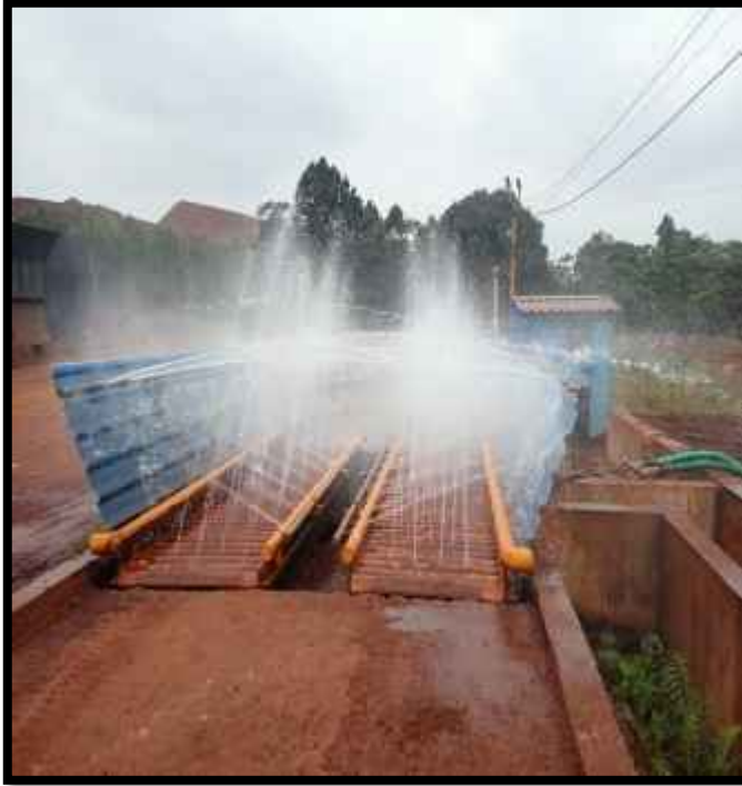
Wheel washing system and Dust suppressant chemical trial
