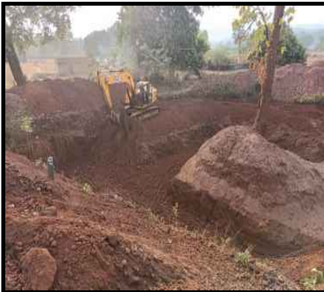
Series of settling pit
