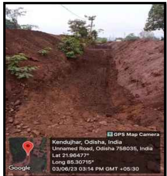
Series of settling pit
