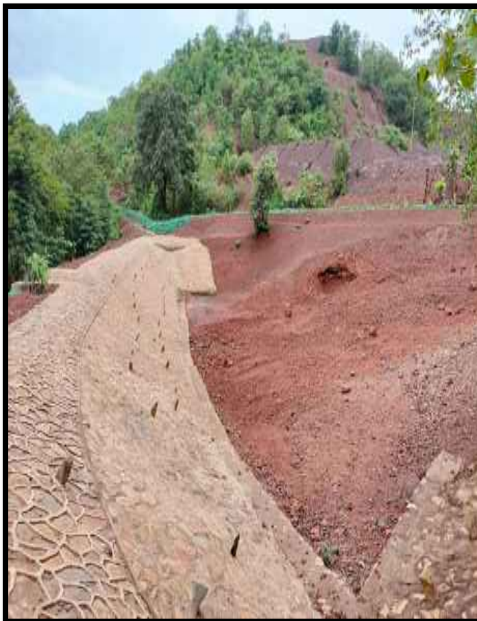
KANHUSAHI RAINWATER HARVESTING OF DIMENSION (50m*60m*2m)
