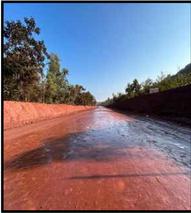
Maintaining ideal haul road width and berm height
