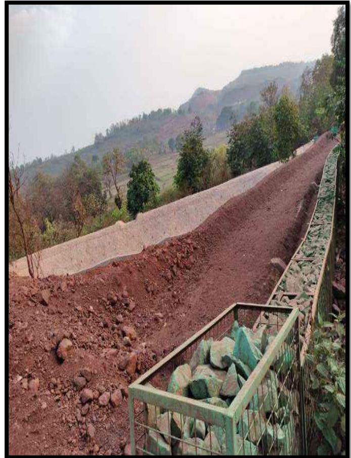
KANHUSAHI RAINWATER HARVESTING OF DIMENSION (50m*60m*2m)
