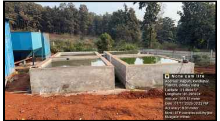
ETP (with Oil Skimmer) and STP (operator colony)
