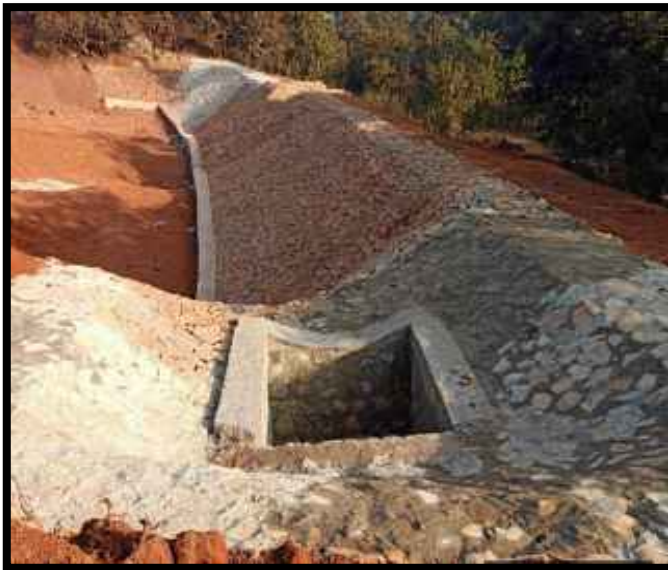
Rainwater harvesting structure at Kanhusahi area
